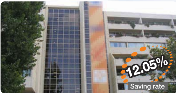
Hospital in Greece U-500
